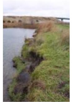
This spring, the Webster County Conservation staff will be laying erosion-control fabric on the shoreline. A private contractor will then haul limestone to be placed on top of the fabric to absorb wave action.
